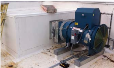
Model TCVSSH Elevator Shaft Exhaust
