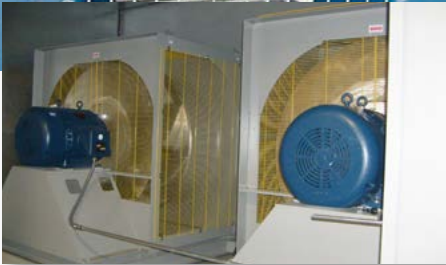
Model EPFN Air Handling Unit
