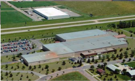
Brookings, SD Manufacturing Facility
