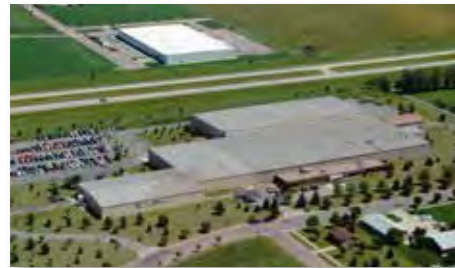
Brookings, SD Manufacturing Facility
